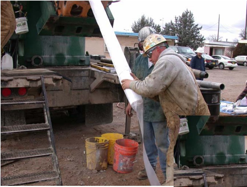
sliding the plastic cover over the NAPL FLUTE cover
